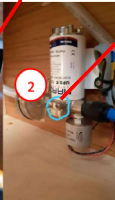
Water pump for tank water supply
